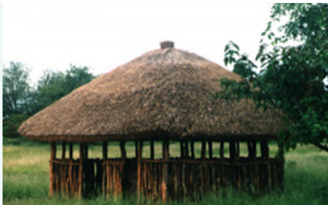
Vetiver based Thatch roof
