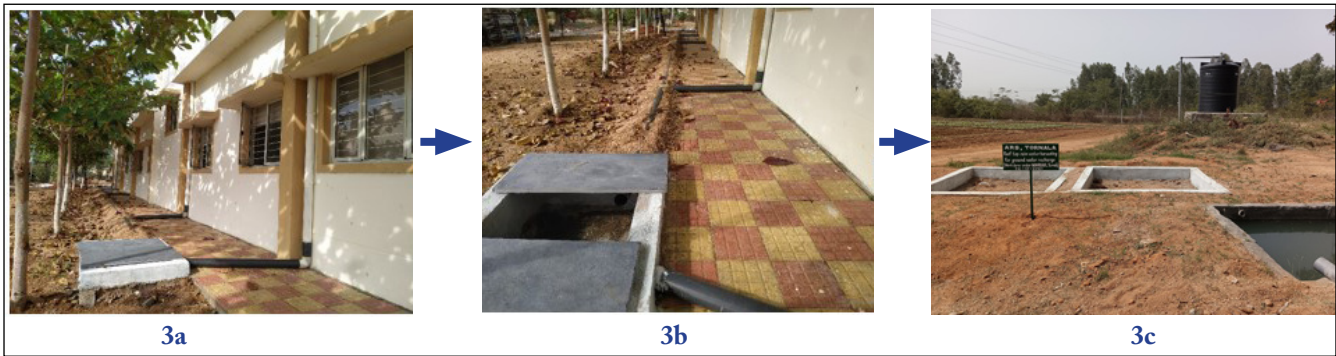
Figure 3: Roof top rain water harvesting for ground water recharge at ARS, Tornala
