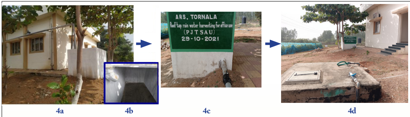
Figure 4: Roof top rain water harvesting for office use at ARS, Tornala
